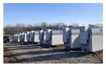
A NEXTracker NX Flow™ integrated solar-plus-storage system. Image: Courtesy of Ideal Energy
