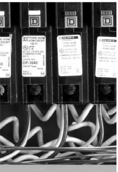
▲ Pigtail Neutral connection
