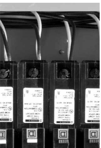
▲ Plug-on Neutral connection
